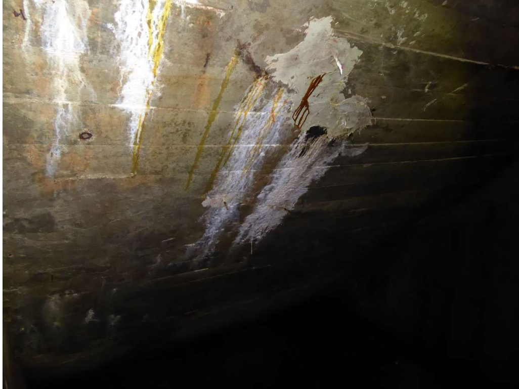
Photo 41: Upstream Face - Chamber #7
