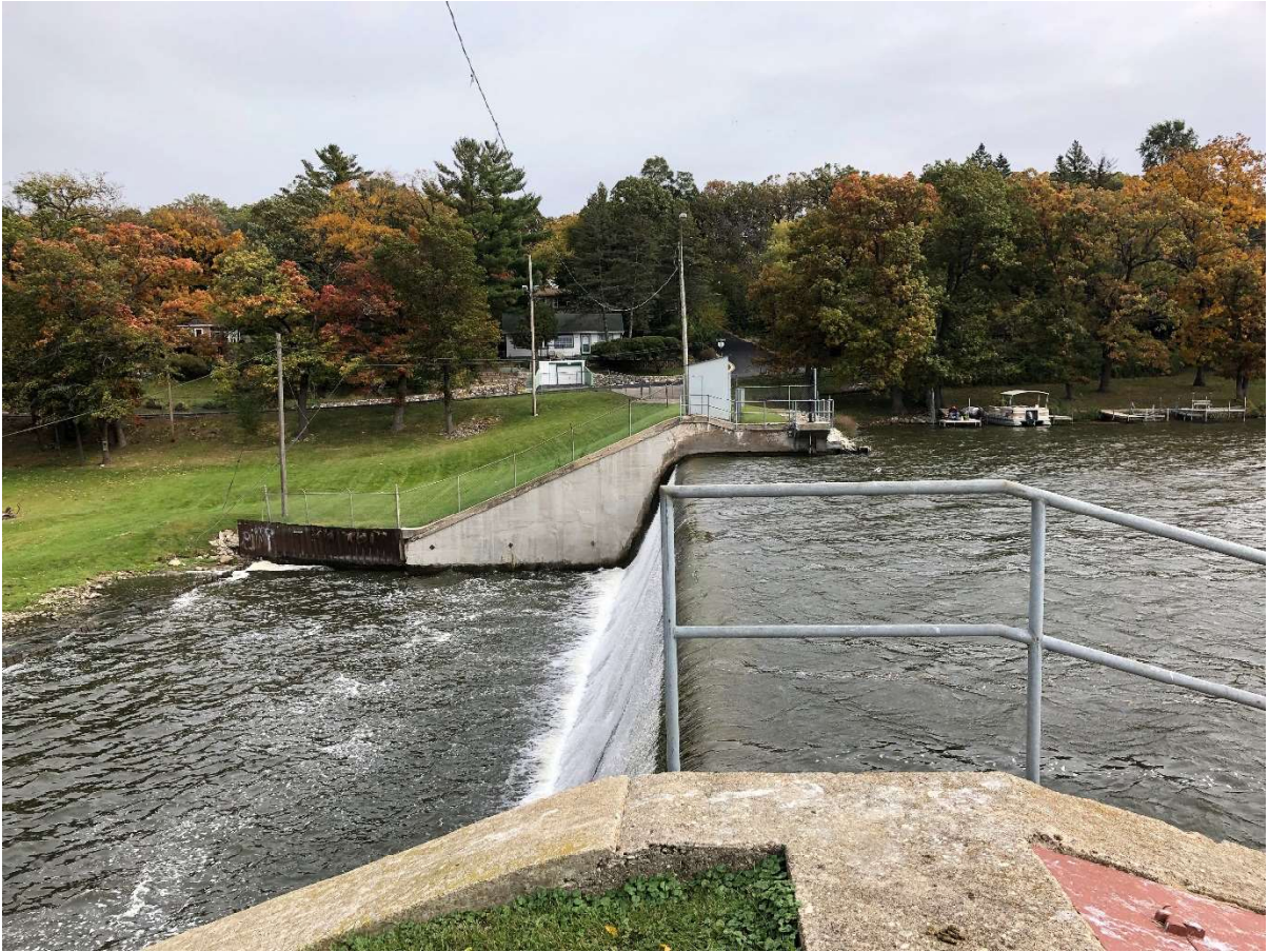
Photo 1: Spillway Crest (Facing east)
