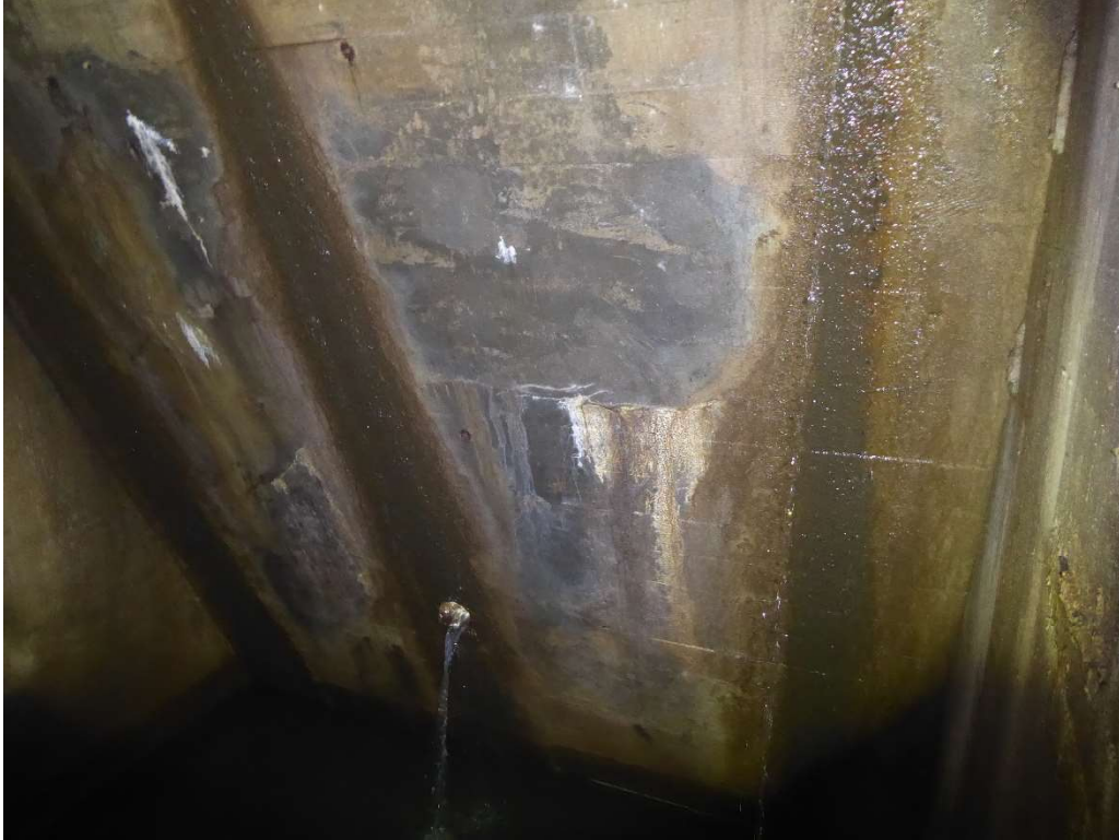
Photo 47: Downstream Wall - Chamber #8
