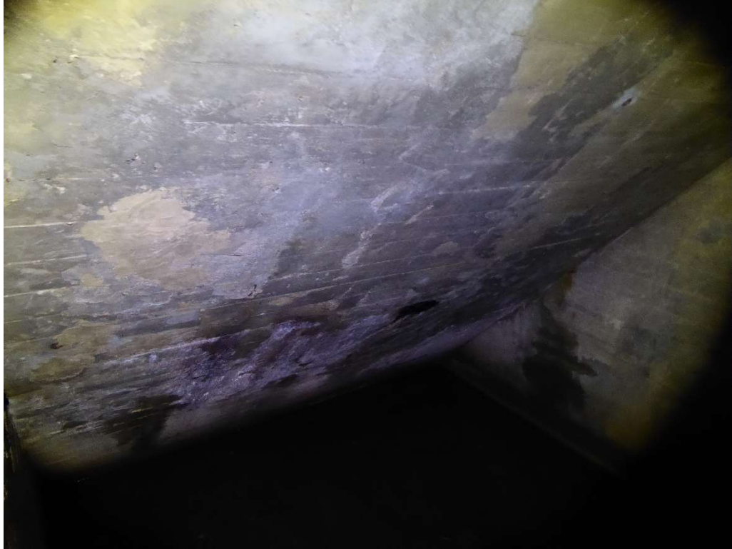
Photo 51: Upstream Wall - Chamber #9
