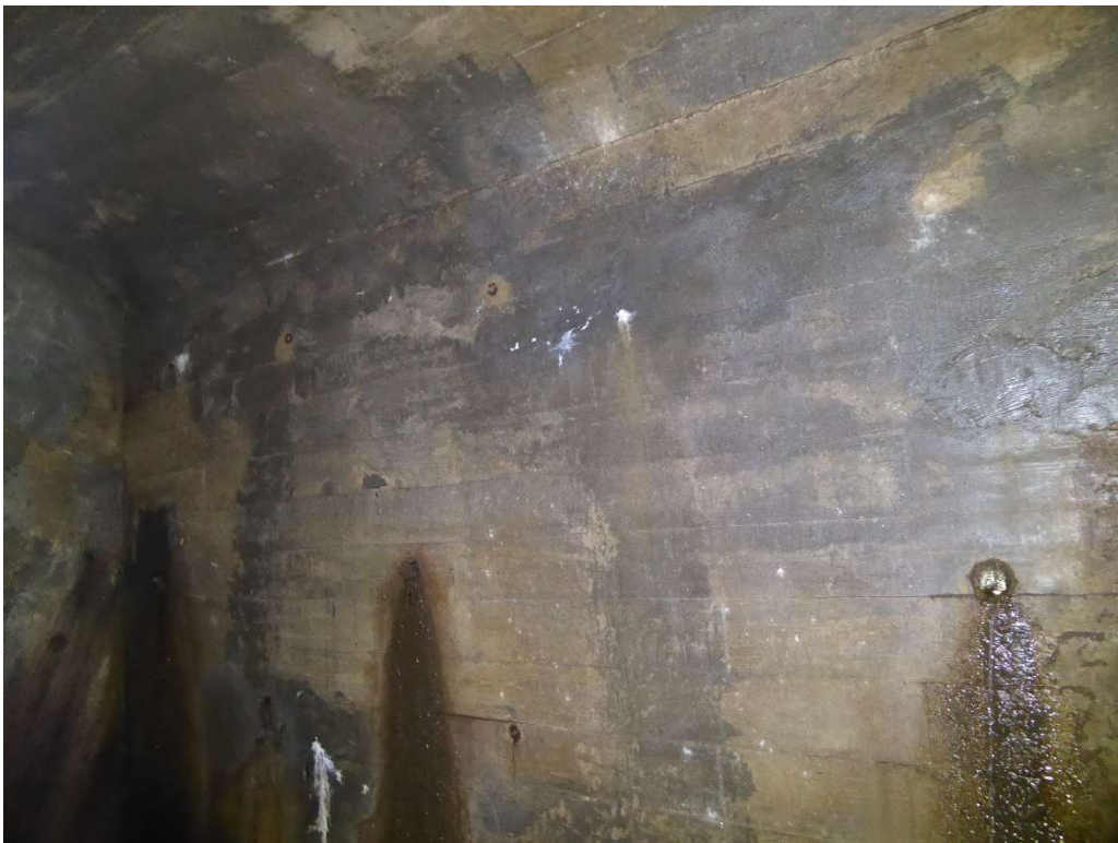
Photo 48: Upstream Wall - Chamber #8
