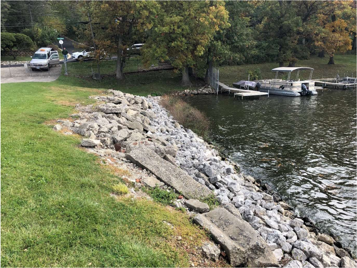
Photo 11: East Embankment – Upstream Face Riprap (Facing East)
