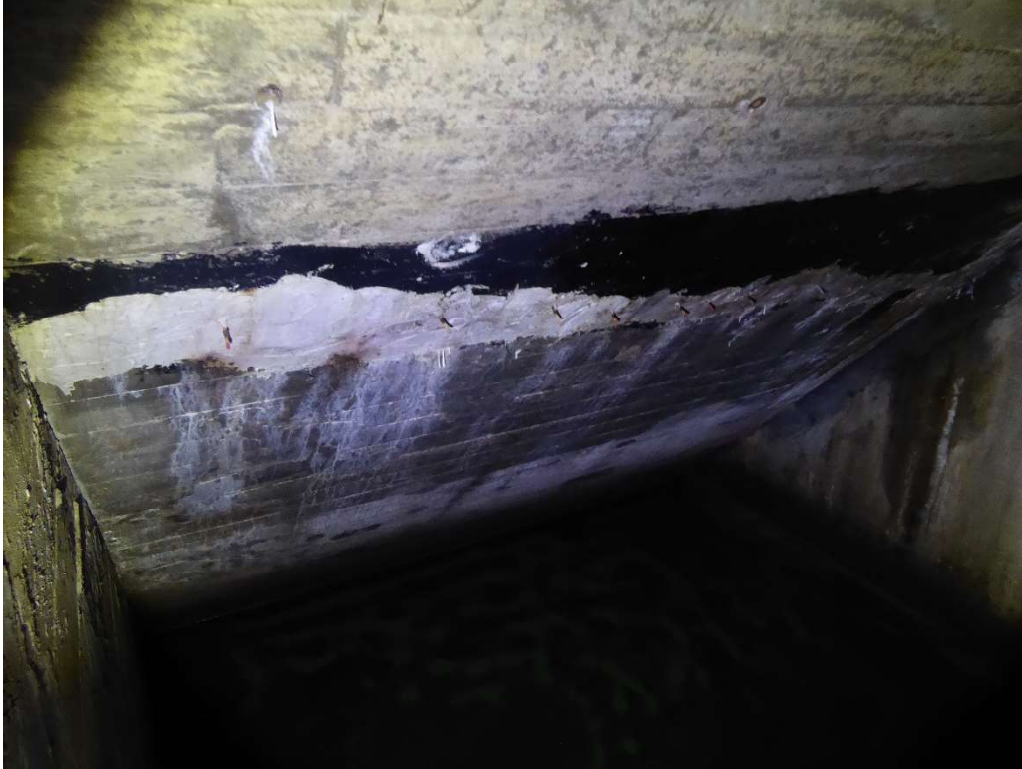
Photo 29: Upstream Face – Chamber #3
