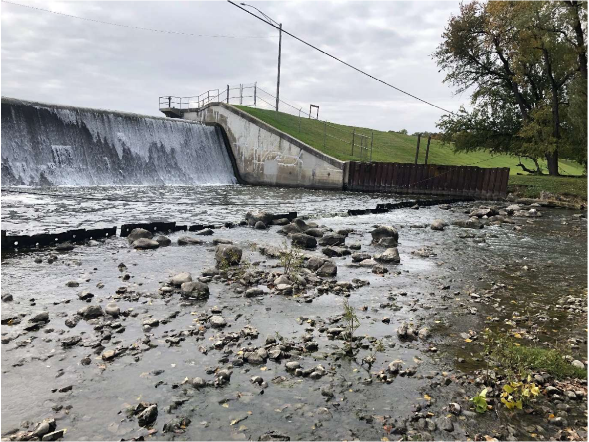
Photo 14: West Spillway Abutment (Facing West)
