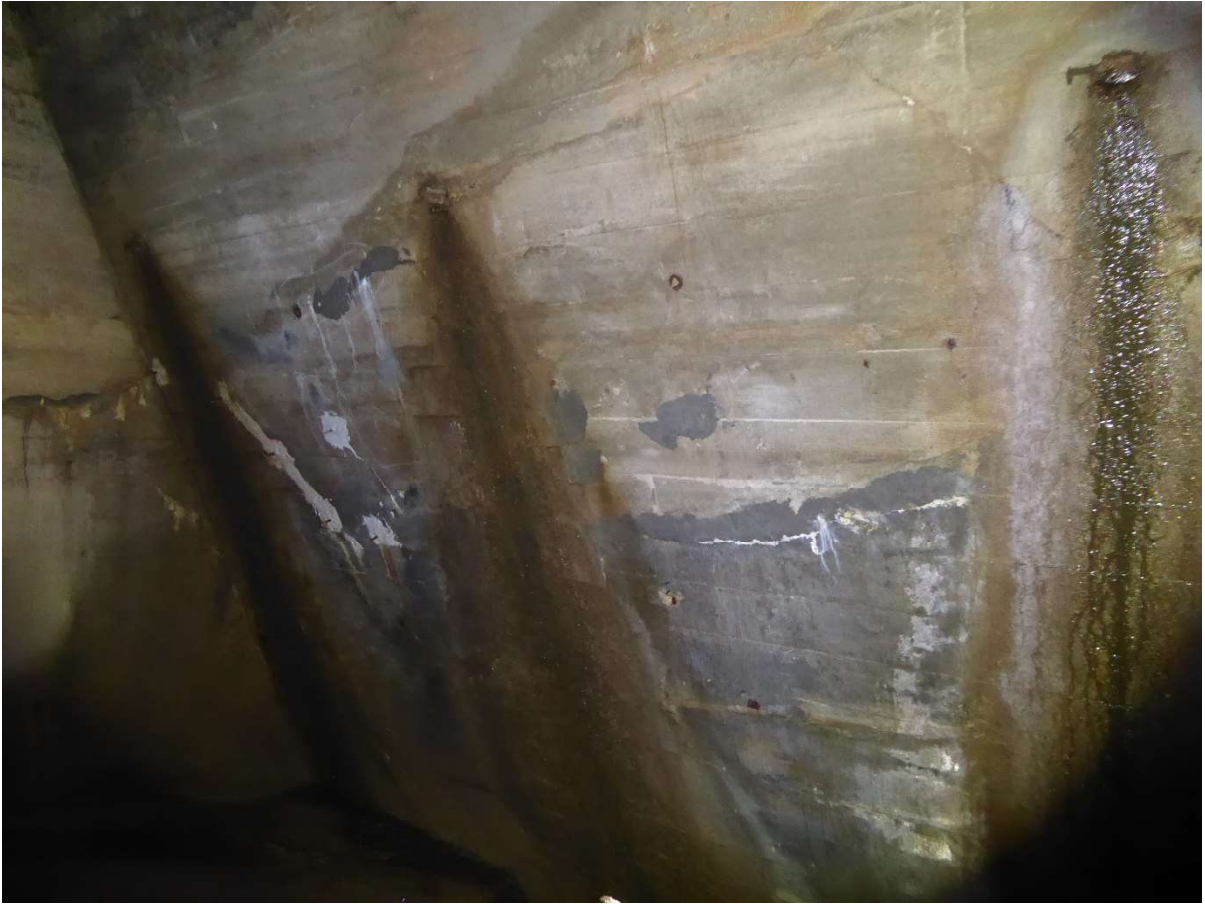
Photo 55: Downstream Wall- Chamber 10
