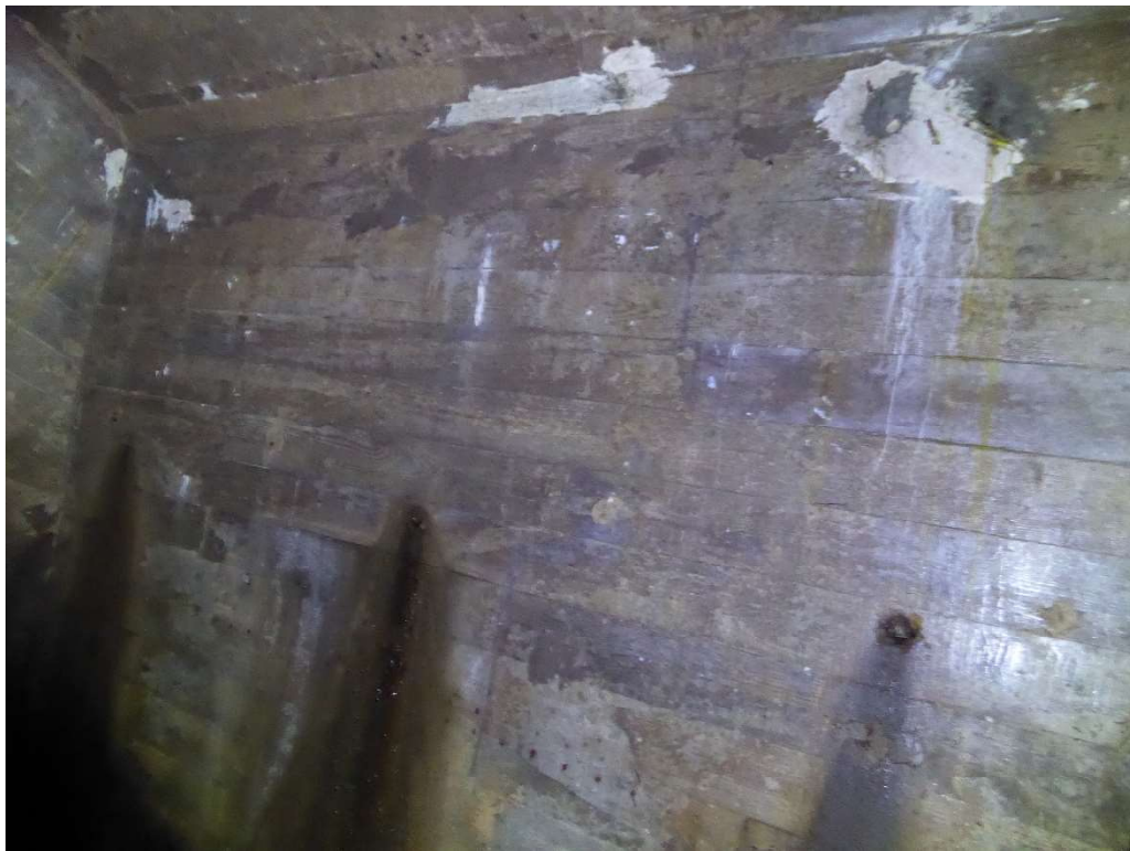
Photo 32: Downstream Face - Chamber #4
