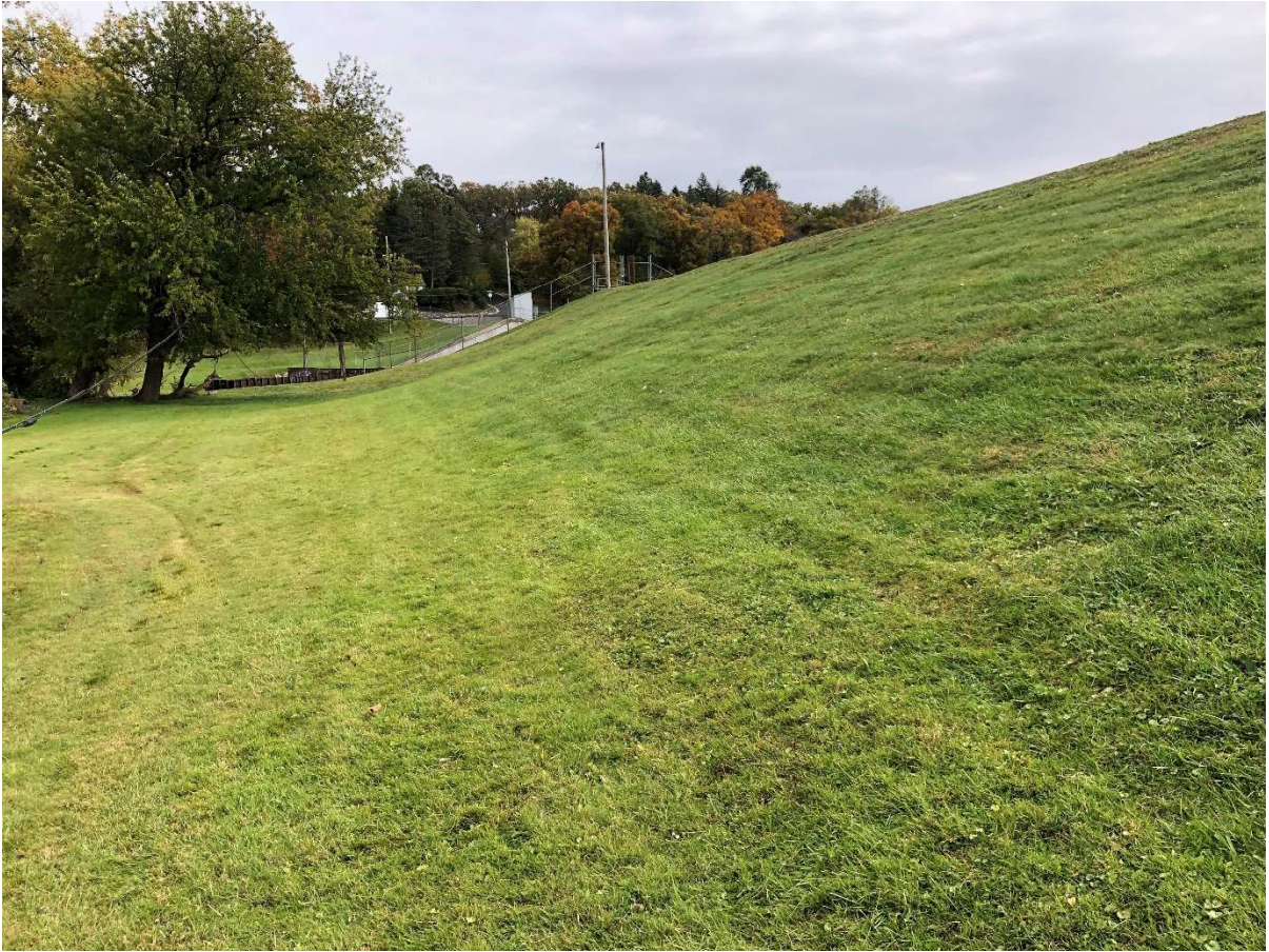
Photo 12: Downstream Side of West Embankment (Facing East)
