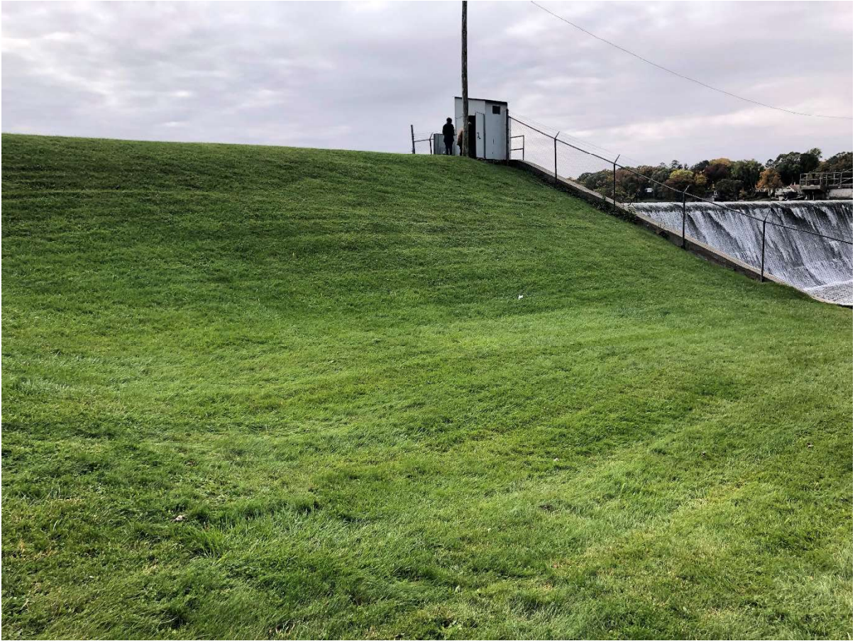
Photo 6: Downstream Face of East Embankment
