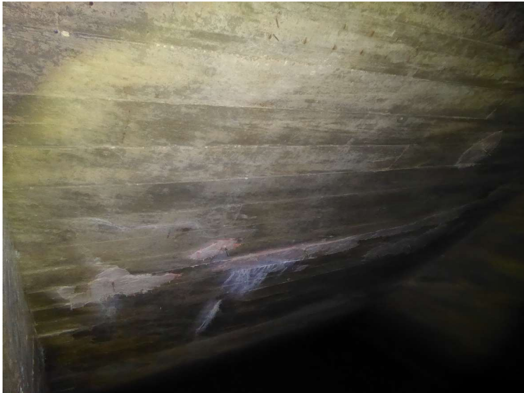
Photo 36: Upstream Face - Chamber #5
