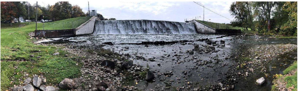
Photo 2: Downstream Face of Spillway
