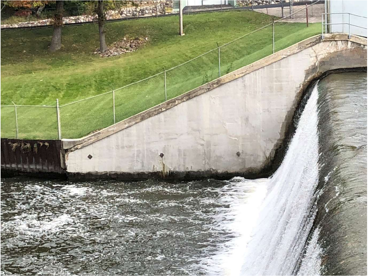
Photo 15: East Spillway Abutment (Facing East)
