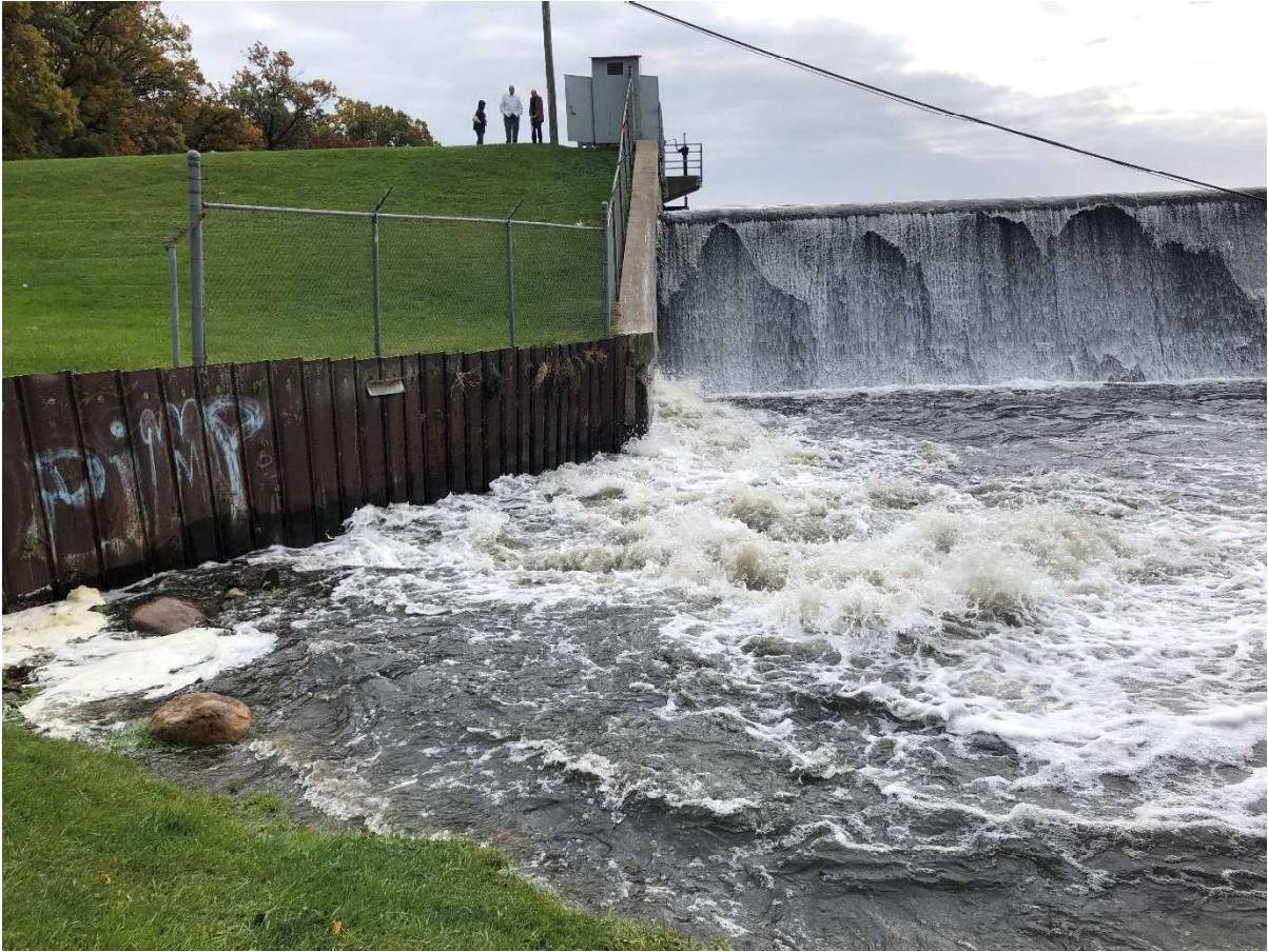
Photo 4 - Downstream Face of Spillway with Sluice Gate Open (East Abutment)
