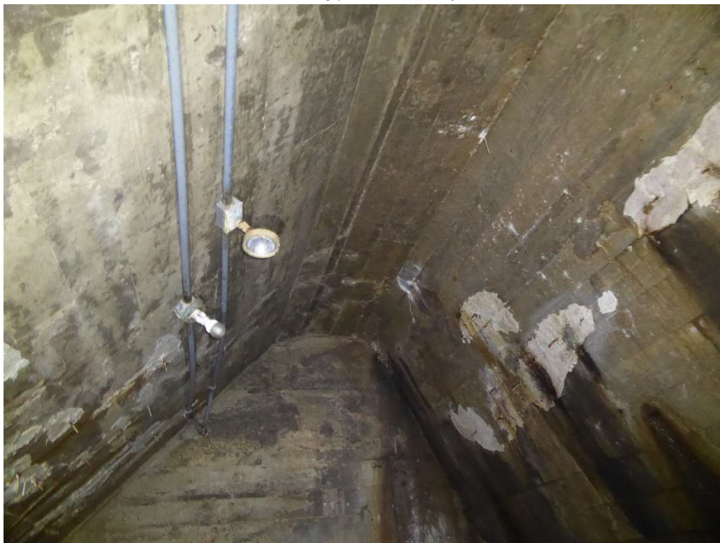
Photo 38: Downstream Face – Chamber #6
