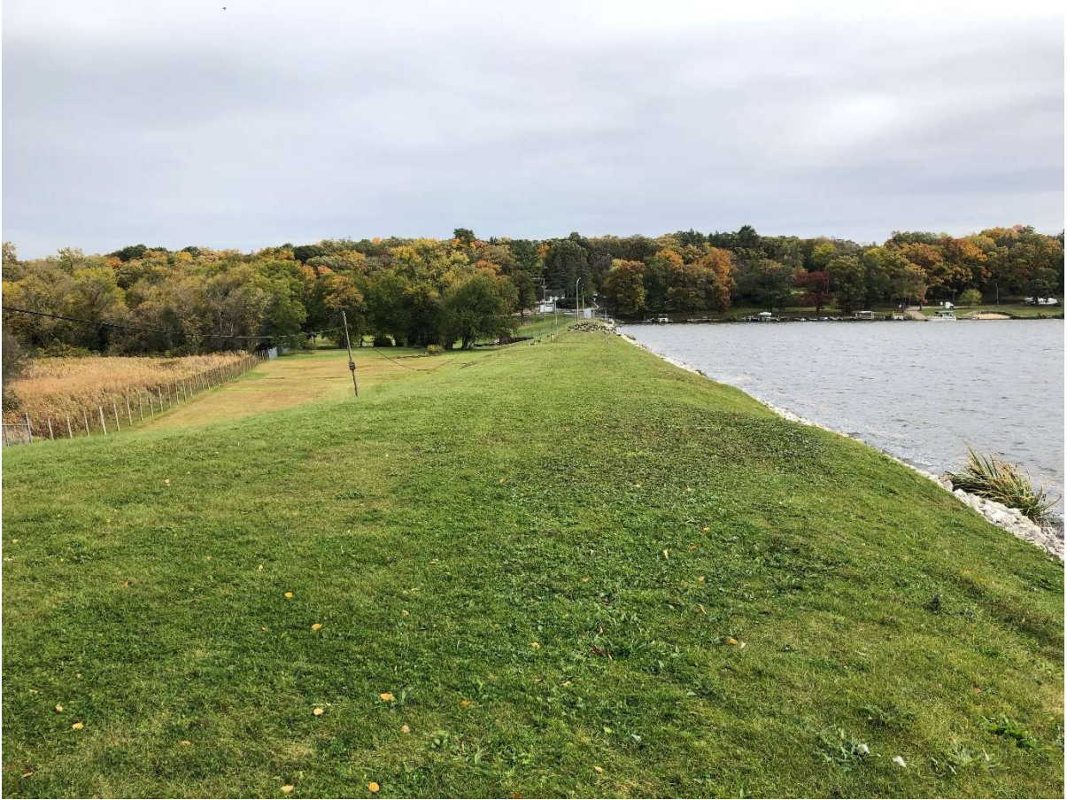
Photo 13: West Embankment (Facing East)
