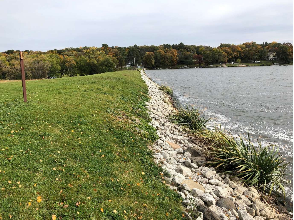
Photo 13: Upstream Side of West Embankment (Facing East)
