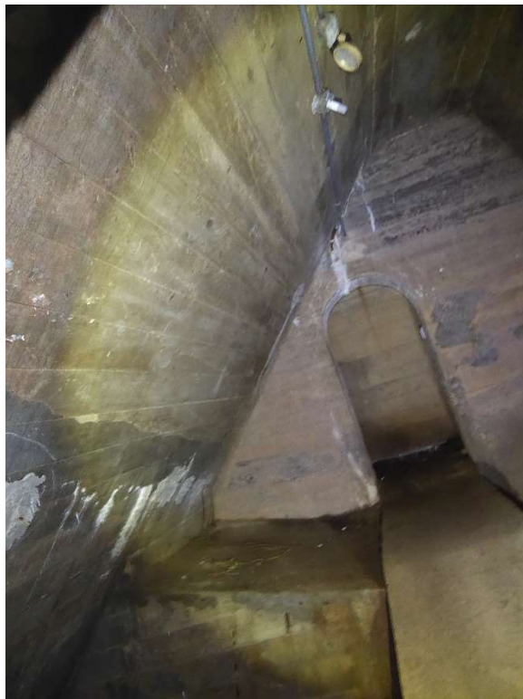
Photo 54: Upstream Wall - Chamber #10
