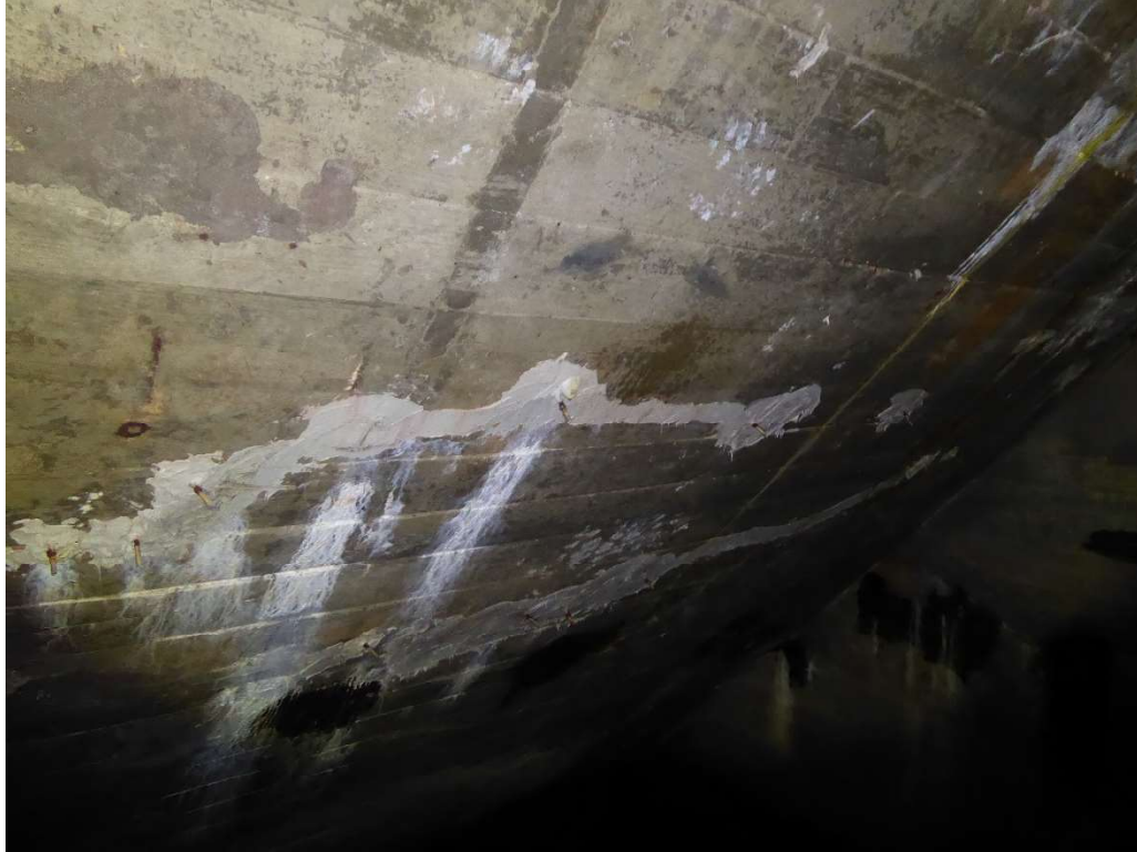
Photo 39: Upstream Face – Chamber #6
