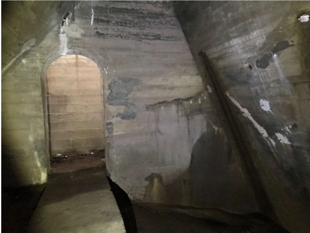
Photo 53: Downstream Wall - Chamber #10
