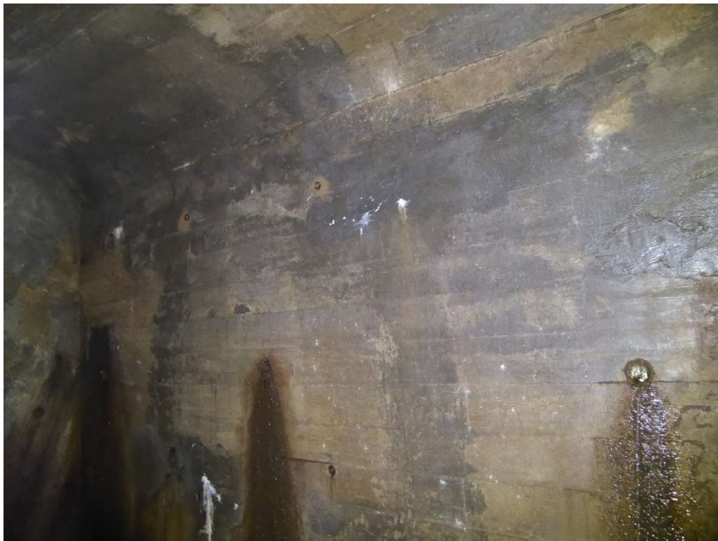
Photo 46 Downstream Wall – Chamber 8
