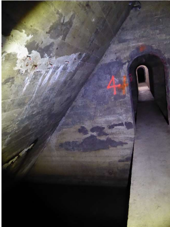
Photo 33: Upstream Face - Chamber #4
