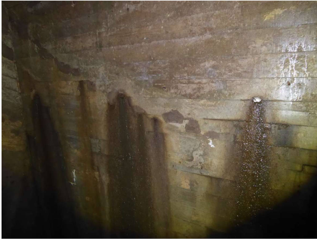
Photo 35: Downstream Face – Chamber #5
