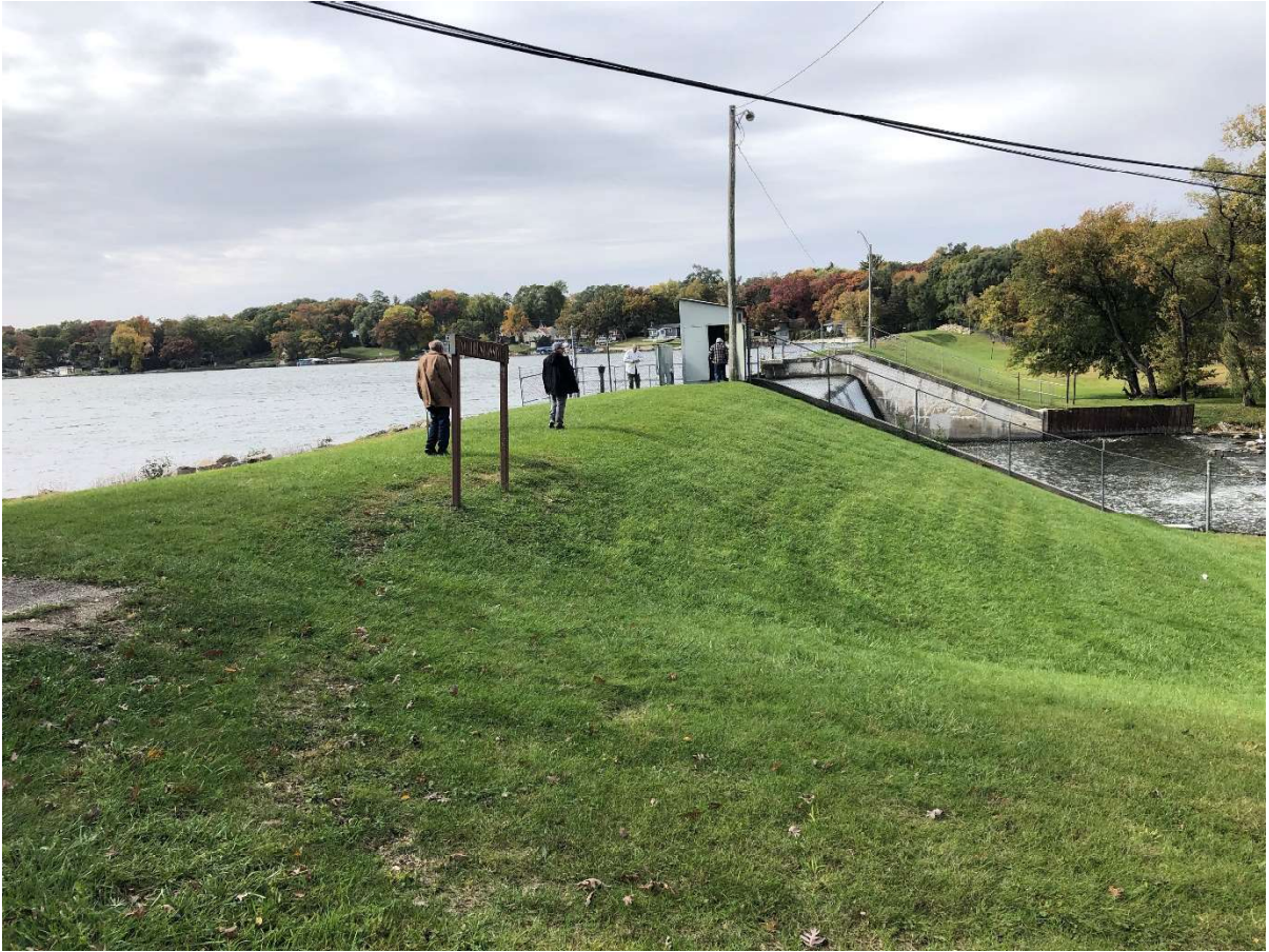
Photo 7: Top of East Embankment (Facing west)
