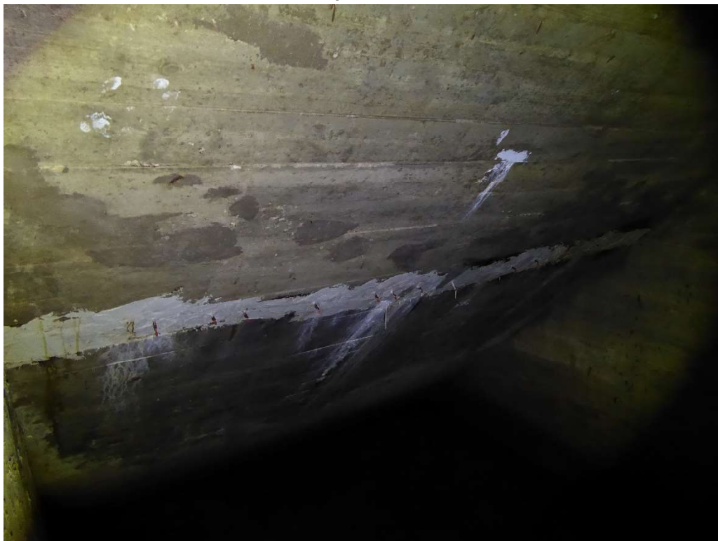
Photo 26: Upstream Wall – Chamber #2
