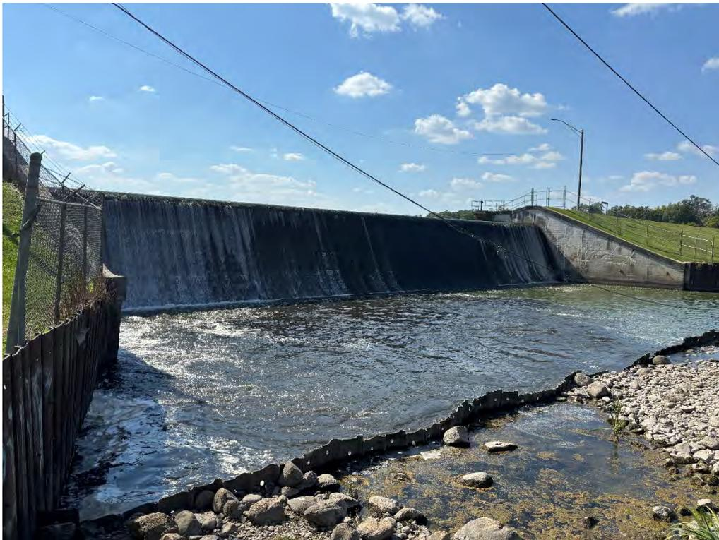
Photo 2: Downstream Face of Spillway
