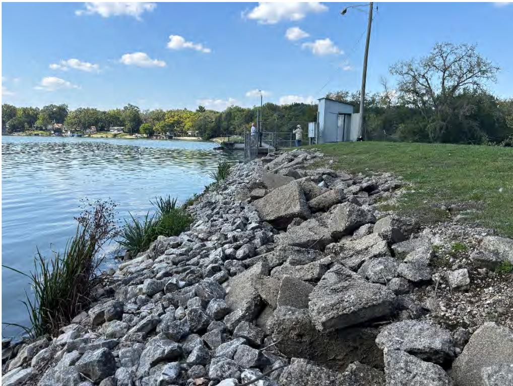
Photo 12: East Embankment – Upstream Face Riprap (Facing West)
